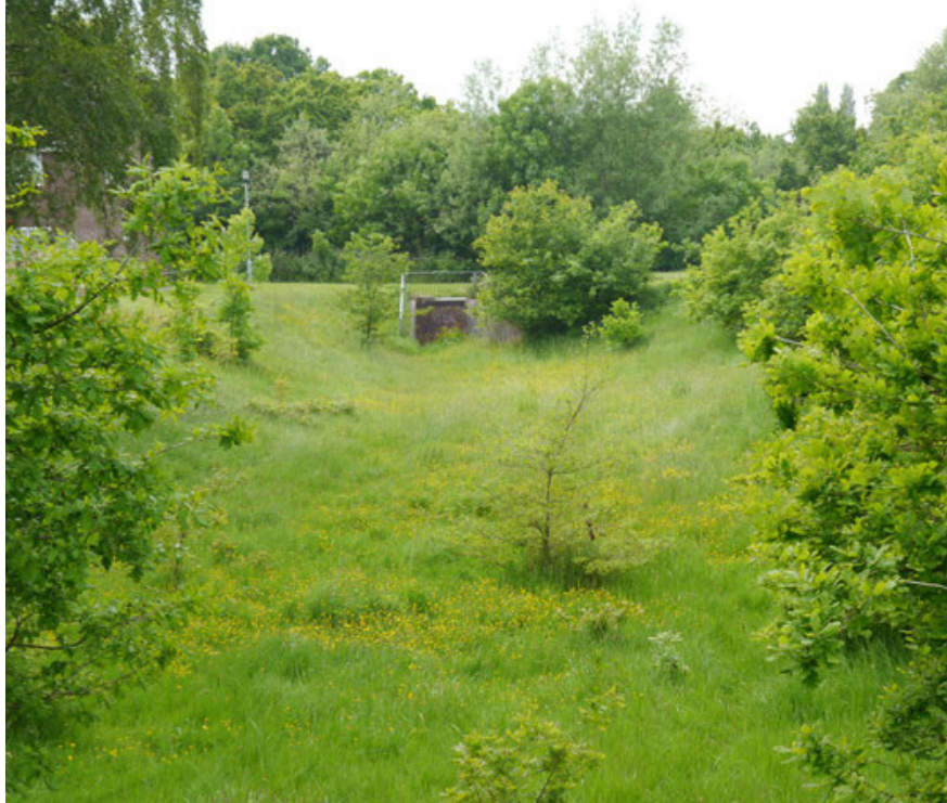
Above ground surface water attenuation pond designed and constructed in the late 1970's/early 1980's – Stockport, Greater Manchester.
